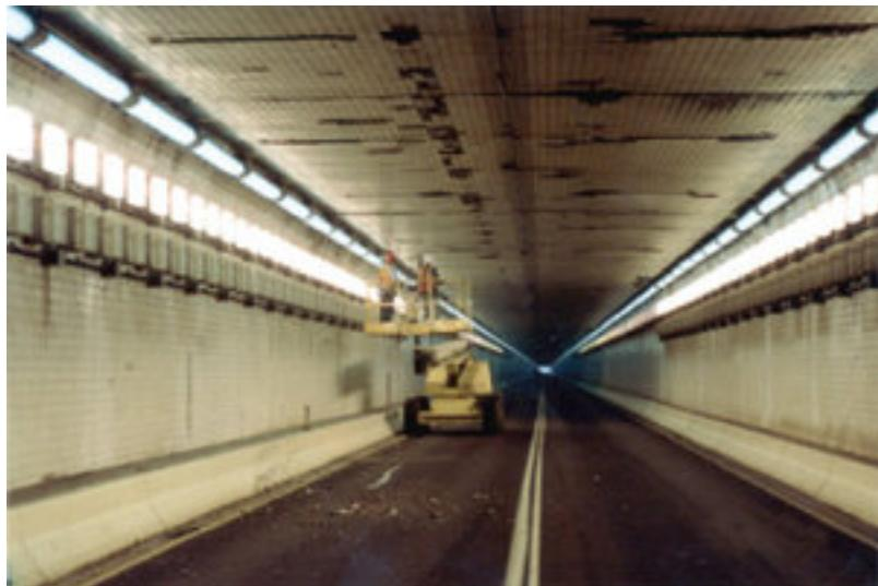
Non-destructive investigations are those undertaken without damage to the lining. They virtually enable to carry out a continuous inspection of a facility and in particular to detect abnormalities that afterwards must be investigated in a destructive way using all appropriate means.
