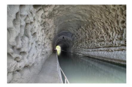
As navigation canals have to be built as horizontal as possible, as soon as topographical accidents appear the construction of tunnels is needed.
