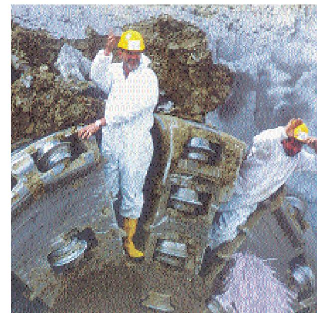
excavation and first-phase segmental lining, designed to withstand TBM and outer rock mass pressures, had to be followed by the placing of a second-phase inner strongly-reinforced concrete shell, in order to resist the inner and outer operational pressures.
