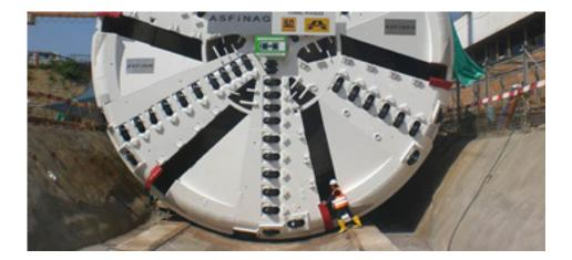
The general principle of the shield is based on a cylindrical steel assembly pushed forward on the axis of the tunnel while at the same time excavating the soil.
