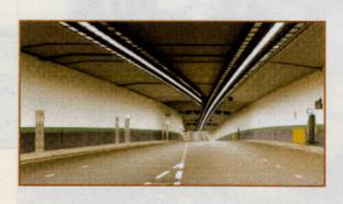
Watertightness: It is often assumed that the process of building a tunnel in water, rather than boring through the ground beneath it will increase the likelihood of leakage. In fact, immersed tunnels are nearly always much drier than bored tunnels, due to the above-ground construction of the elements. Underwater joints depend on robust rubber seals which have proved effective in dozens of tunnels to date.
